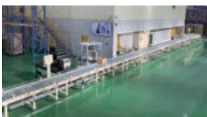
E Plant : E-Beam Irradiation Facility
